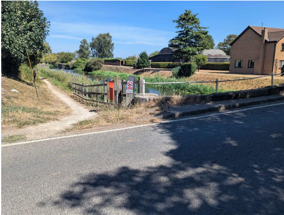
Figure 20. Tankards Bridge 2020 – The Grade II listed bridge parapet was badly damaged by a large vehicle – due to the damage the Canal and River Trust had to close the Aire to Selby Canal for several months while awaiting bridge repair due to the risk to boat traffic. The road was then also closed for several days in 2021 while final permanent repairs were completed.
