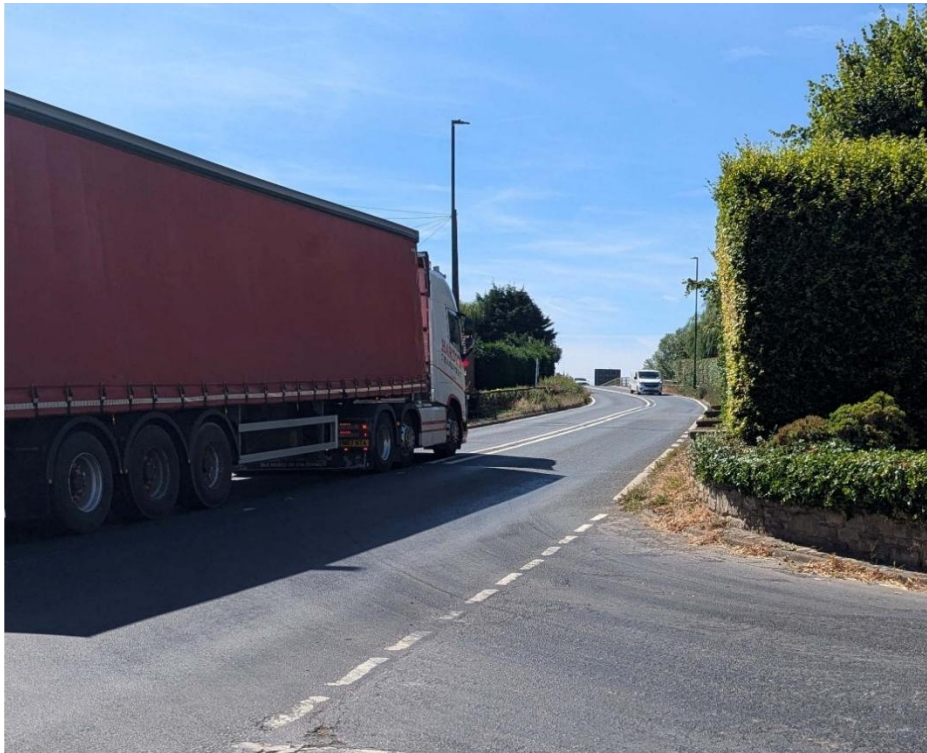
Figure 3. View from Millfield Road looking south to the Aire Bridge – note short distance from brow of bridge to turning point
