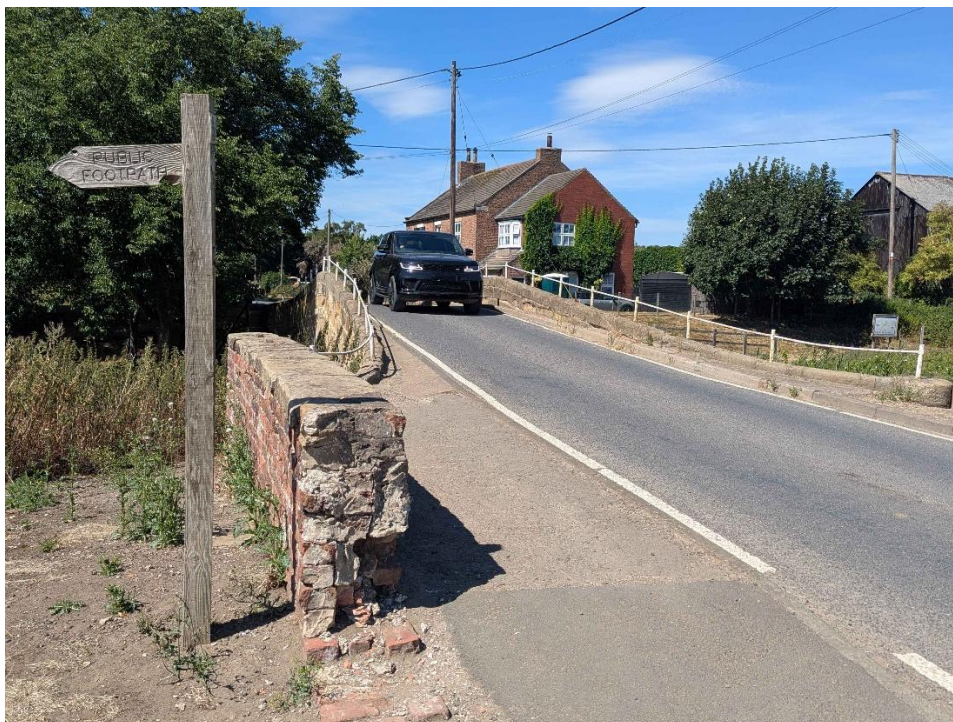
Figure 18. Grade II listed, single lane, Tankard's Bridge showing one of the two public footpaths at the bridge (the other footpath being to the right along the canal on the other side of the bridge – see next photo), absence of footway on bridge and single lane over the canal.
